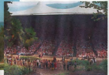
Living example of longevity: The grand stand of the open-air theatre in Elspe (D), realized in 1978 with Type IV PVC-coated membrane by Mehler Technologies.
