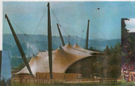
Living example of longevity: The grand stand of the open-air theatre in Elspe (D), realized in 1978 with Type IV PVC-coated membrane by Mehler Technologies.
