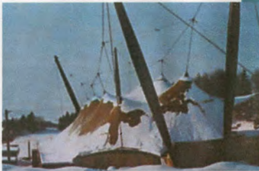
Living example of longevity: The grand stand of the open-air theatre in Elspe (D), realized in 1978 with Type IV PVC-coated membrane by Mehler Technologies.
